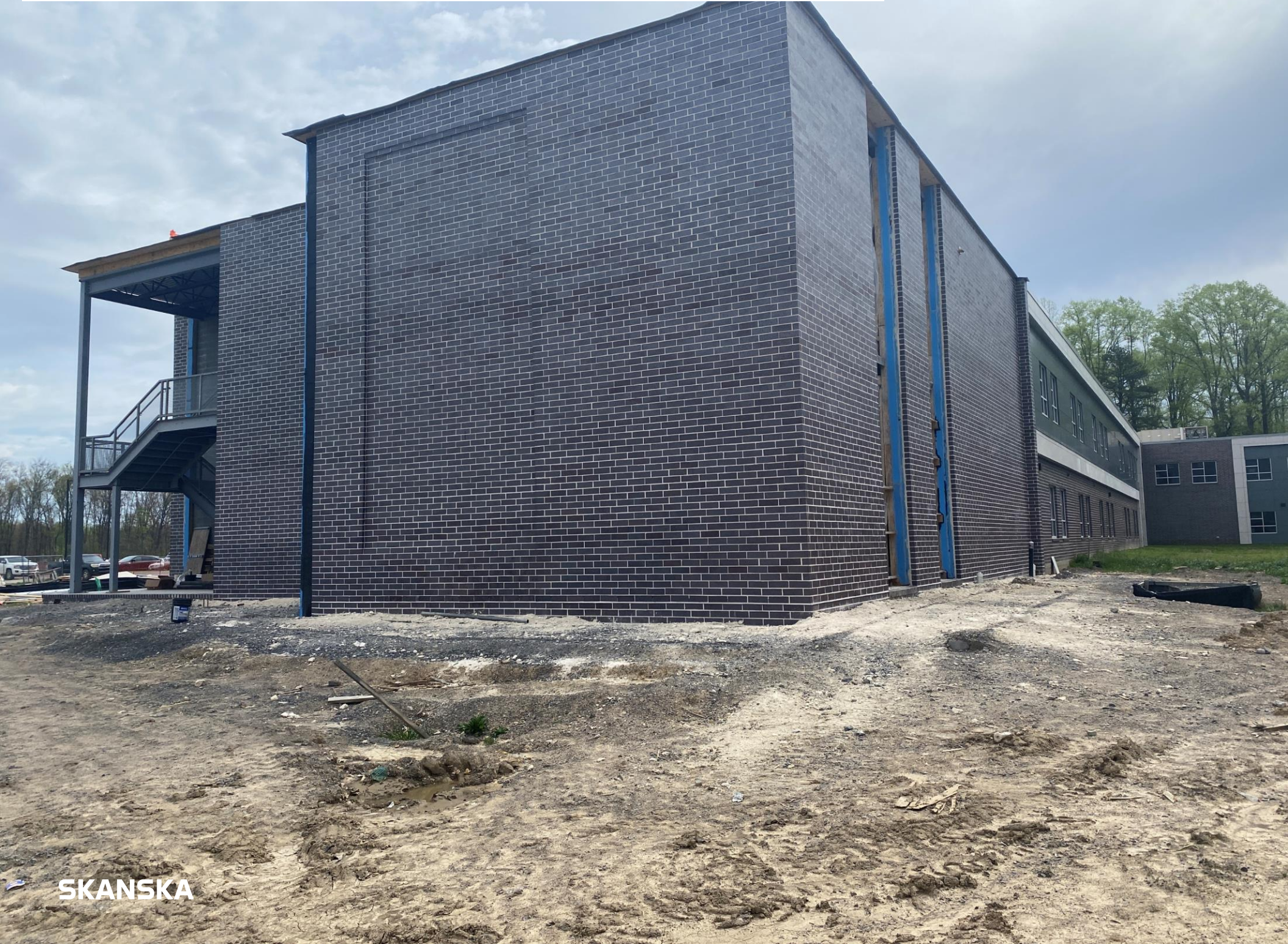
Southwest corner of new addition – brick installation complete
